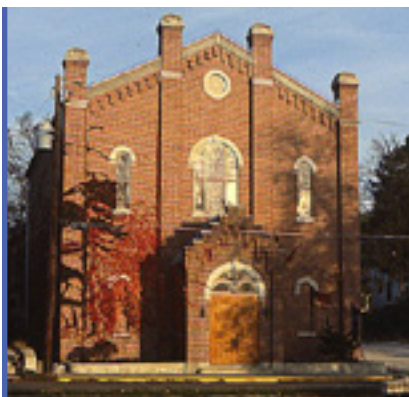
Fellowship members restored the former Temple Israel in Lafayette, now listed on the National Register of Historic Places.
